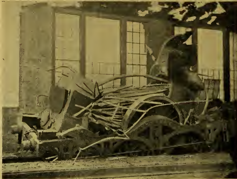
SINGLE-DRIVER BROAD-GAUGE LOCOMOTIVE "PERSEUS," G.W.R., AFTER EXPLOSION OF BOILER.
