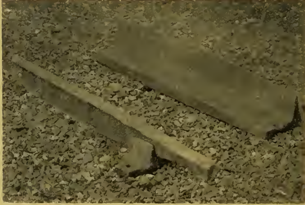
BRANCH LINE RAIL AND CHAIR, AND MAIN LINE TRAM PLATE, KILMARNOCK & TROON RY.
