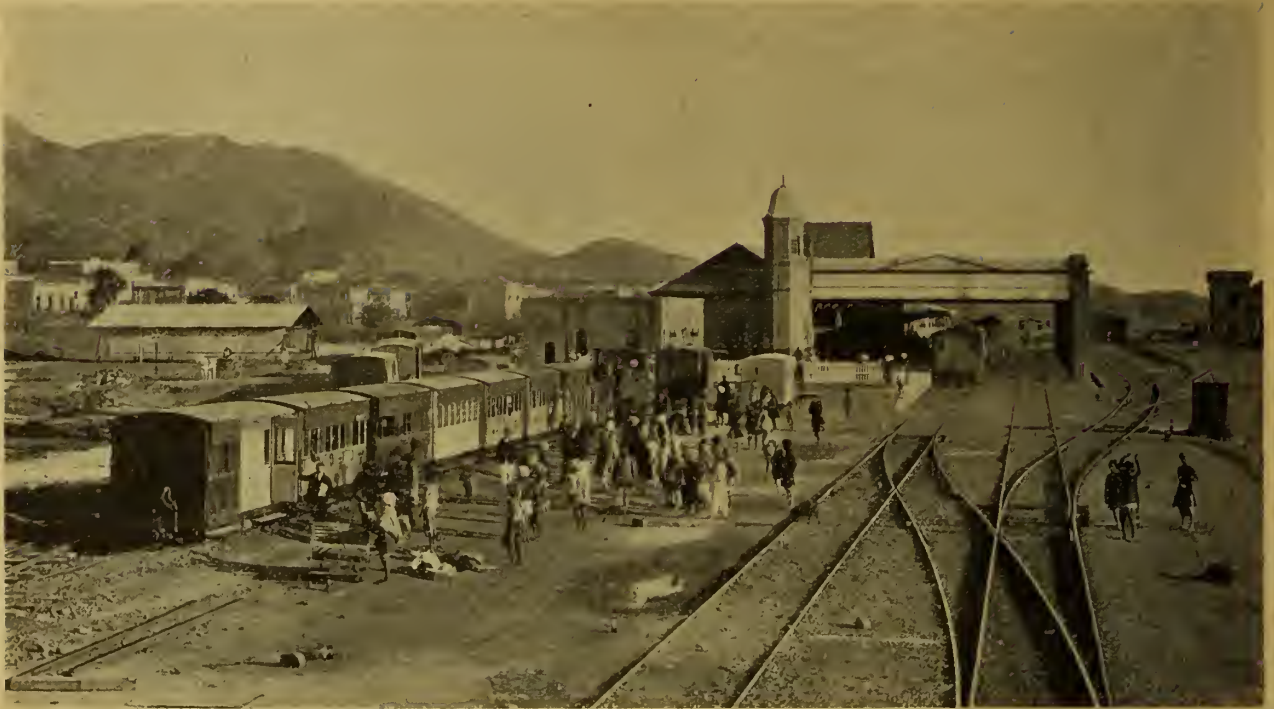
KALKA JUNCTION STATION, SHOWING NARROW-GAUGE TRAIN, KALKA-SIMLA RY.
