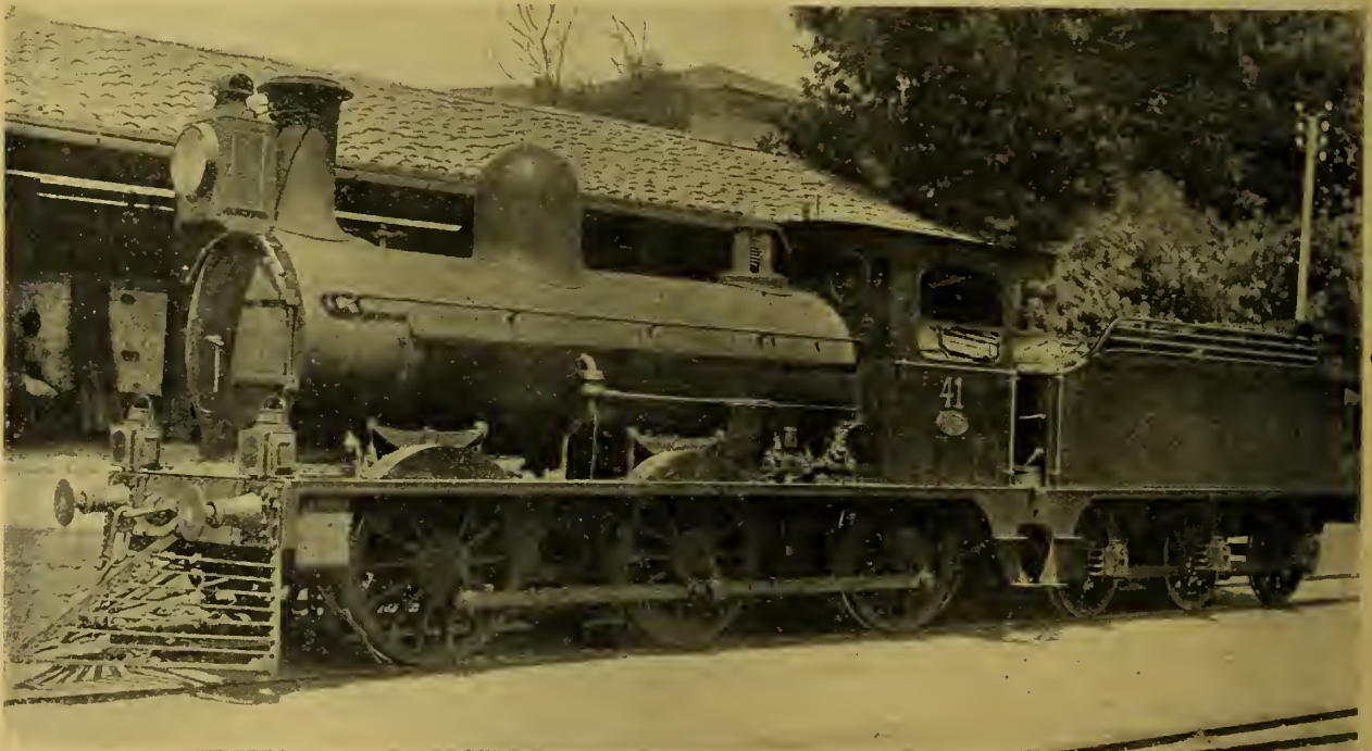
SIX-WHEELS COUPLED GOODS LOCOMOTIVE No. 41 (No. 4 CLASS), OTTOMAN (AIDIN) RY.
