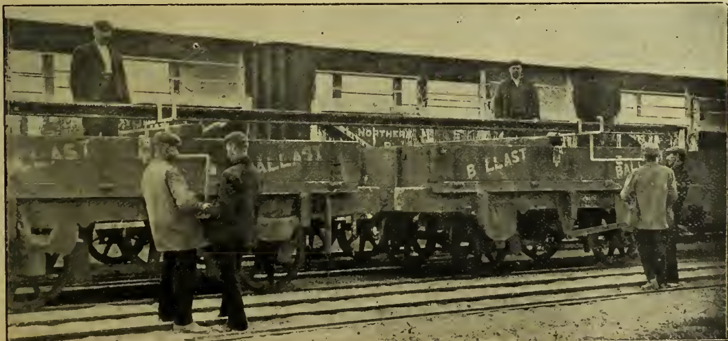
FIG. 2.—RAIL LOADER IN OPERATION : RAIL LIFTED ON TO CROSS SUPPORTS OF WAGONS.
