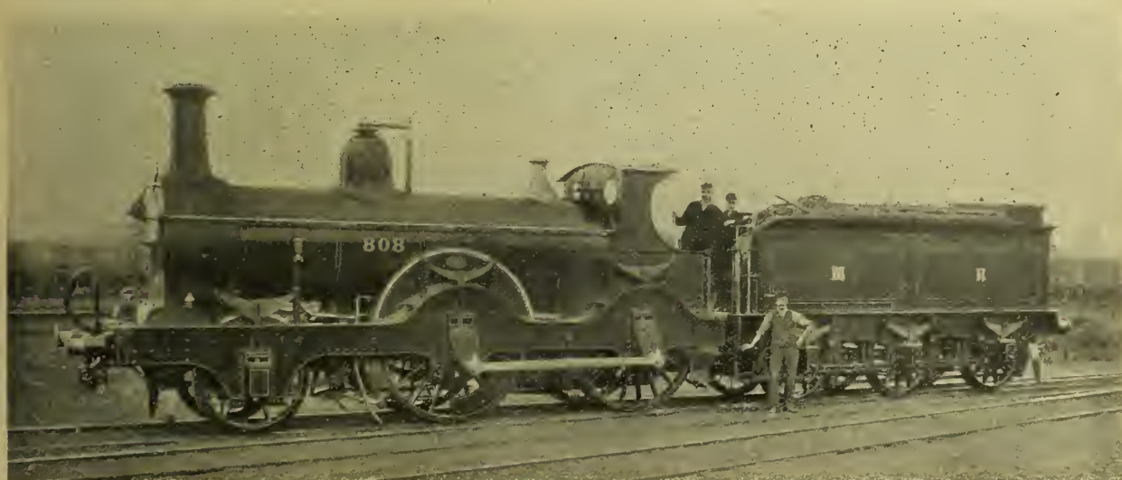
FOUR-WHEELS COUPLED PASSENGER LOCOMOTIVE NO. 808, AS REBUILT, MIDLAND RY.
