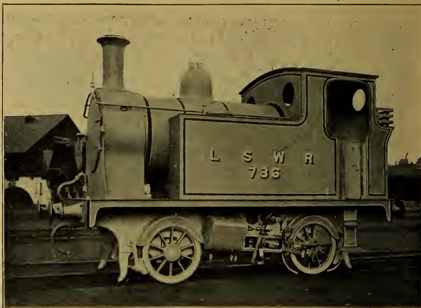
STEAM MOTOR LOCOMOTIVE No. 736, LONDON & SOUTH WESTERN RY.
