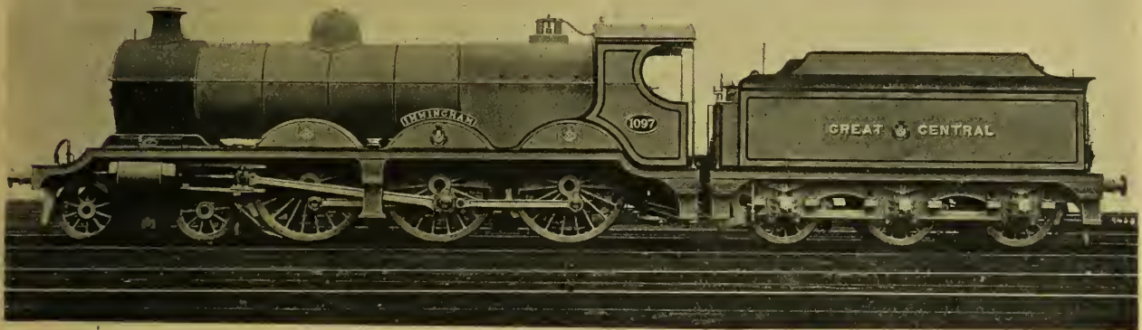
SIX-COUPLED BOGIE PASSENGER EXPRESS LOCOMOTIVE No. 1097 "IMMINGHAM," GREAT CENTRAL RY.
