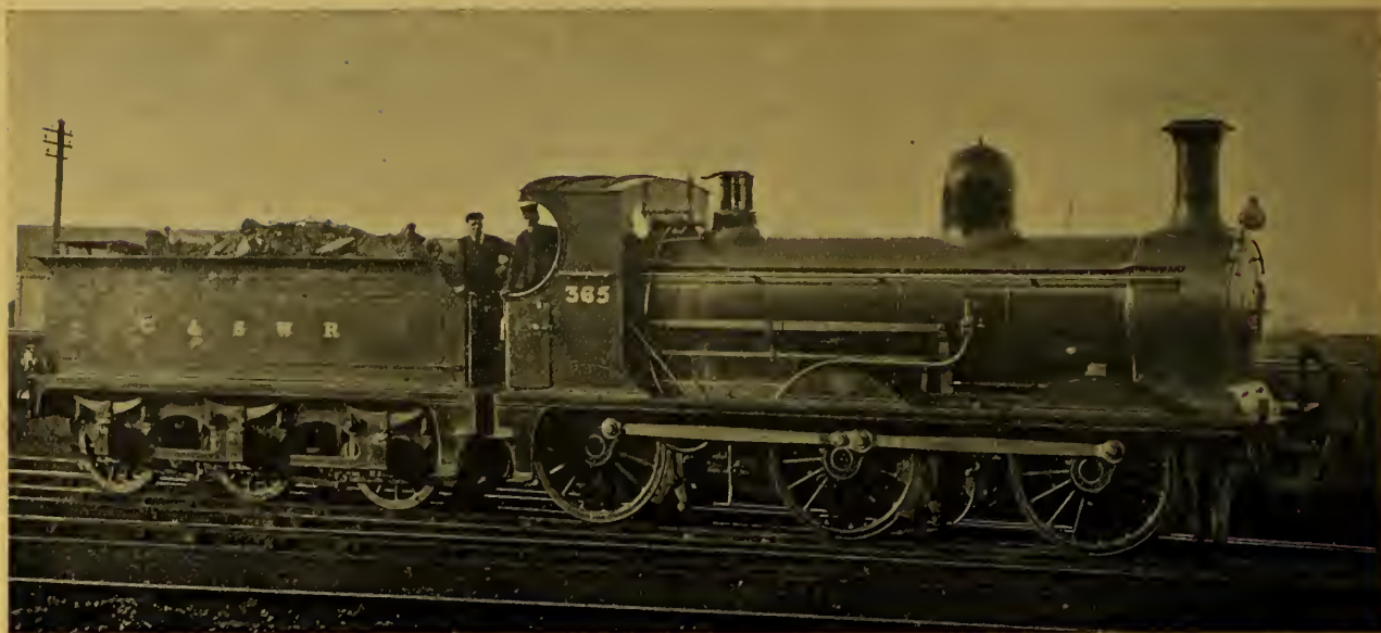
SIX-WHEELS COUPLED GOODS LOCOMOTIVE, No. 365, GLASGOW &amp; SOUTH WESTERN RY.
