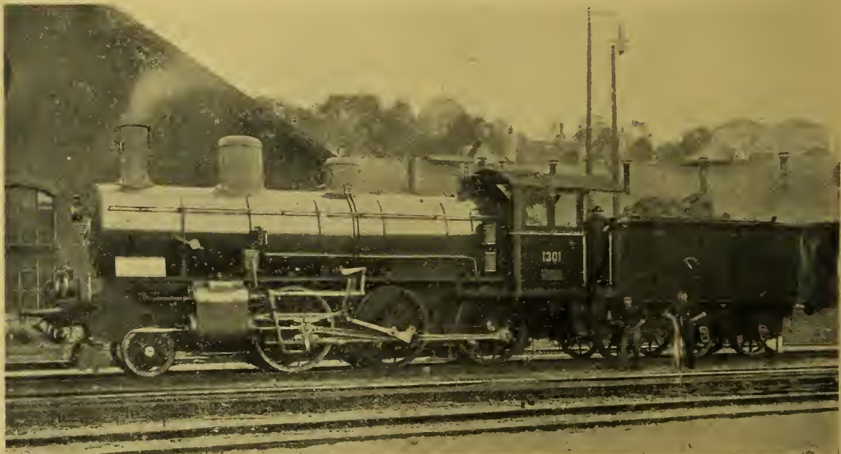
MOGUL LOCOMOTIVE No. 1301, CLASS B 1 1/2 , WITH SCHMIDT SUPERHEATER, SWISS STATE RYS.
